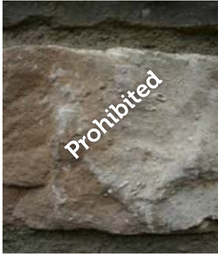
Unnatural looking stone from a worn out mold with poor detailing example
