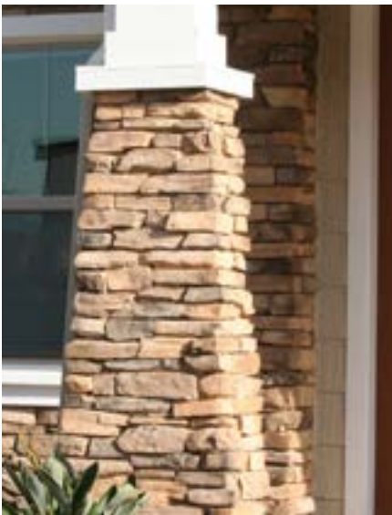
Examples of veneers wrapping columns entirely
