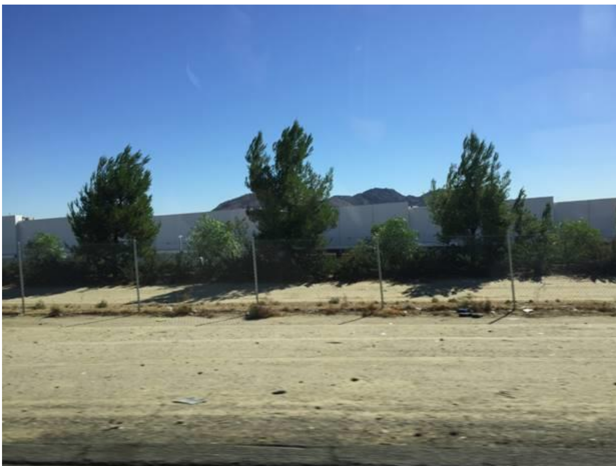
View of Existing Skechers Building from SR-60 Eastbound
