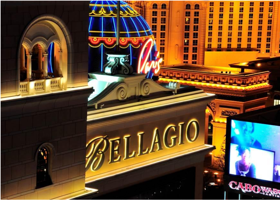
Bellagio Resort Hotel & Casino • Las Vegas, Nevada 37 Story - 3,015 Rooms & 8-Level Parking Garage 48 Traction Elevators • 23 Hydraulic Elevators • 16 Escalators • 4 Moving Walks Architects: Marnell Corrao Associates • DeRuyter O. Butler Architect Service Type: New Facility Design
