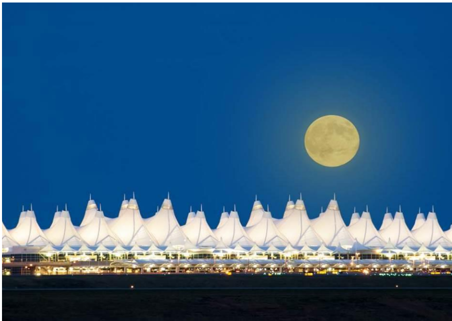
Denver International Airport • Denver, Colorado Six Level Main Terminal Building - Approximately 1,350,000 GSF Four Level Parking Structure - Approximately 3,100,000 GSF Office Building - Approximately 175,000 GSF 43 Traction Elevators • 10 Hydraulic Elevators • 36 Escalators • 4 Moving Walks Architect: Fentress Bradburn Architects Ltd. Service Type: New Facility Design
