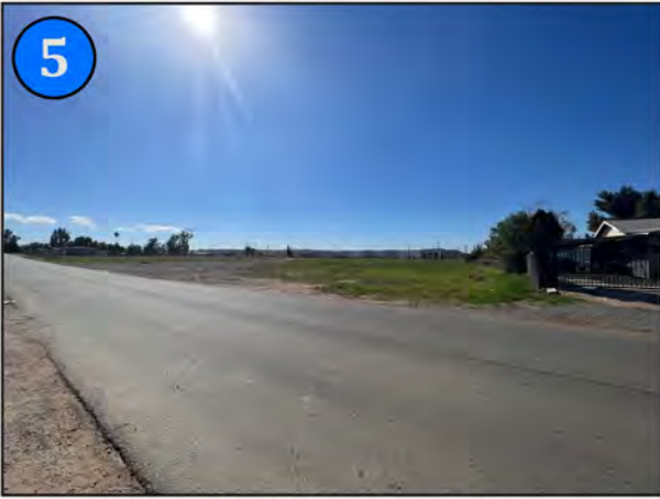
View 5: Northeast of the Project Site along Edgemont St. looking southwest.
