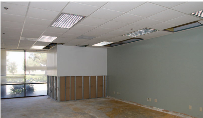
Annex 1 Building Space “Before”
