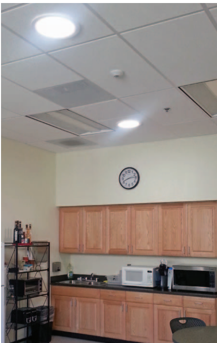
Annex 1 Break Room “After” with Solar Lighting Tubes Installed
