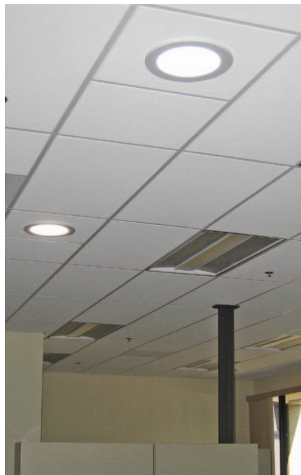
Annex 1 Office Space “After” with Solar Lighting Tubes Installed
