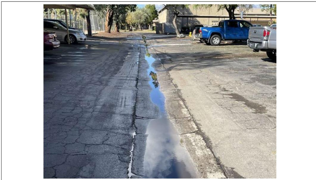
Photo 8: View facing west along the southernmost street along the tennis courts. View of ponded stormwater typically observed throughout Parcel A from recent storm event.
