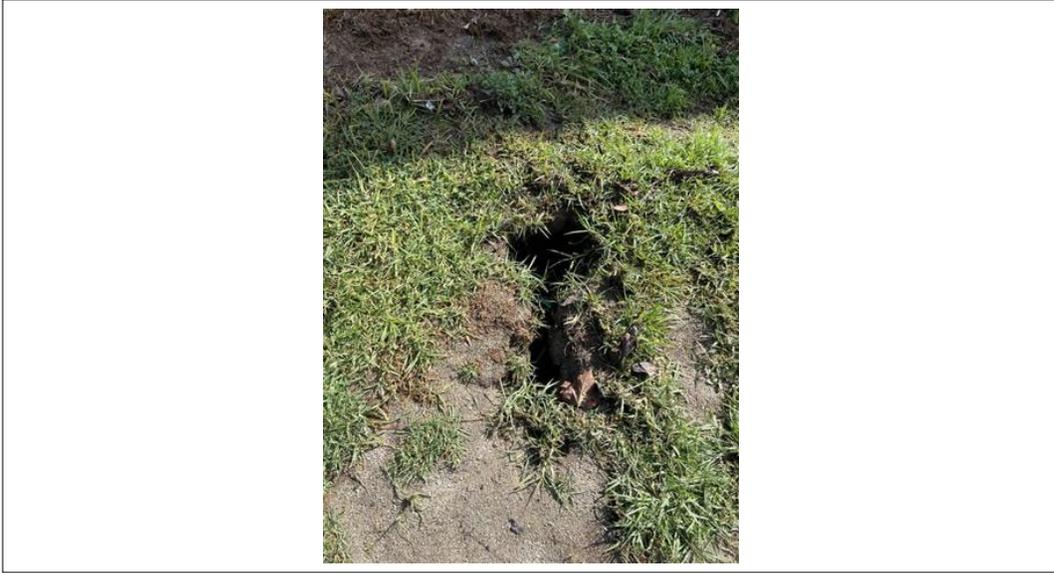
Photo 13: Close up view of a hole in ground/void in the vegetation adjacent to stormwater drainage culvert (see next photo) at north part of Parcel A.
