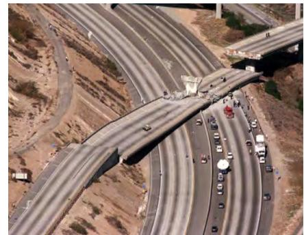
Examples of typical effects of seismically induced ground shaking. The photograph on the left shows a damaged building from the 1994 M6.7 Northridge Earthquake. The building has essentially fallen backwards, and what was once a straight wall now appears curved. The photograph on the right shows the collapsed portion of a freeway overpass from the same earthquake.
