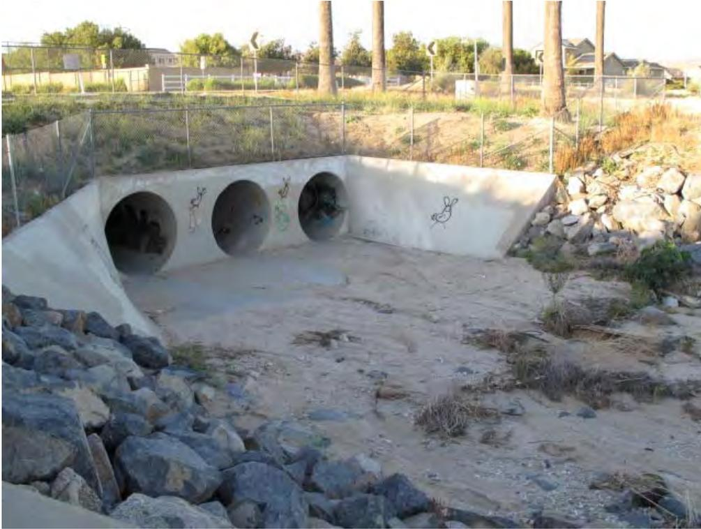
7) Concrete drainage culvert at adjacent stormwater channel.
