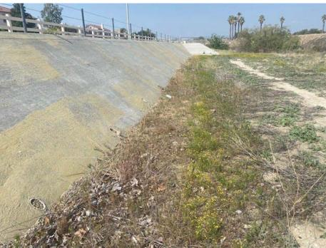
Photograph 31: Weep holes at the base of a concrete flood control wall on the west side of the channel.
