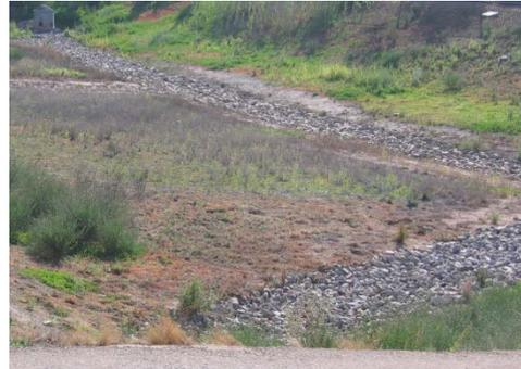
Figure 3: Gravel filled low-flow trench
