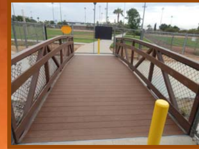
Sunnymead Park ADA Pedestrian Bridge
