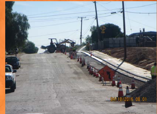
Elsworth Street and Sherman Avenue Sidewalk Improvements
