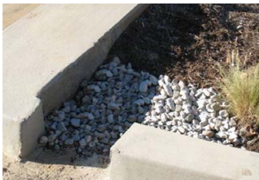
Figure 2: Curb Cut located in a Bioretention Facility
