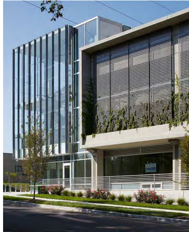
Commercial uses fronting a parking structure to hide the visual impact of the structure.
