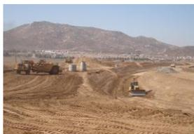
Construction work for the widening and extension of Cactus Avenue and Nason Street is currently on schedule with 10% completion. Clearing/grubbing, remedial
